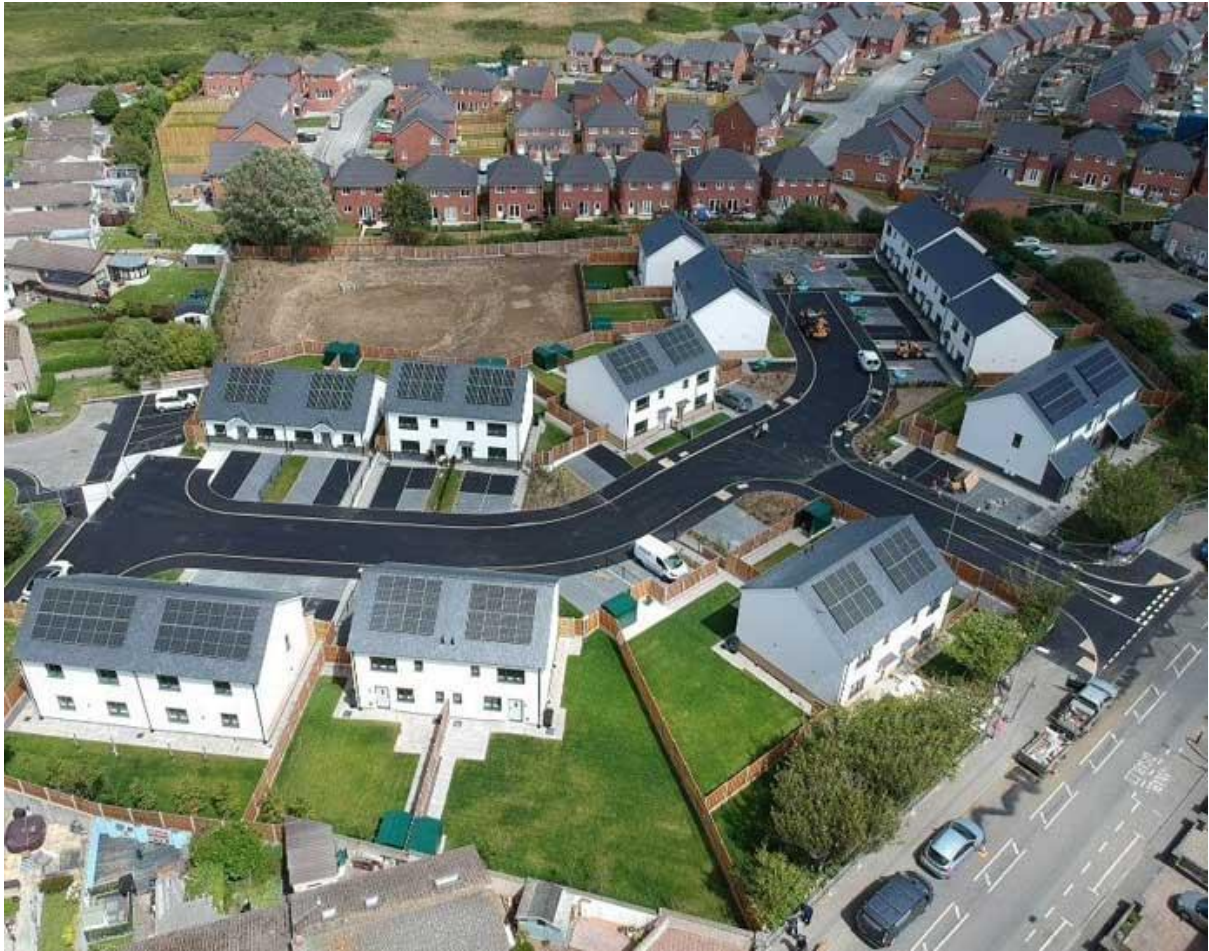
Llaingoch housing development, new estate completed July 2022- Holyhead
